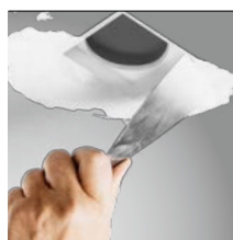
skimmed into plasterboard ceiling (trimless)
