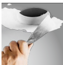
skimmed into plasterboard ceiling (trimless)
