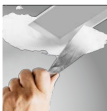
skimmed into plasterboard ceiling (trimless)
