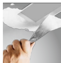
skimmed into plasterboard ceiling (trimless)
