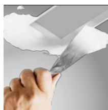
skimmed into plasterboard ceiling (trimless)
