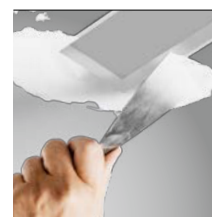
skimmed into plasterboard ceiling (trimless)
