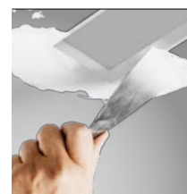
skimmed into plasterboard ceiling (trimless)
