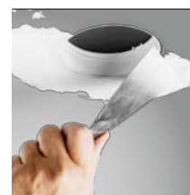
skimmed into plasterboard ceiling (trimless)
