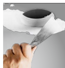
skimmed into plasterboard ceiling (trimless)
