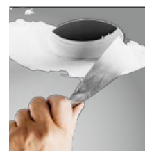
skimmed into plasterboard ceiling (trimless)
