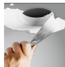
skimmed into plasterboard ceiling (trimless)
